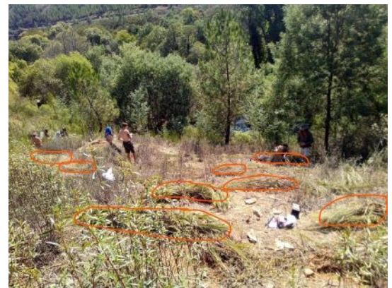
Figure 3: Some of the infiltration ditches (highlighted with orange ellipses) built as part of the workshop organized by EcoAtivo
